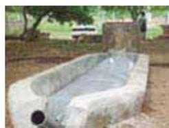
3. A small hole (about one centimetre in diameter) is punctured through the wall of the digester about 1 metre from the inlet end. A small piece (about 30-cm long) of the normal PVC water pipe (1.2
