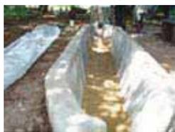
2. The two sides of the digester are fitted with the 4" PVC pipes measuring about 1 m to serve as inlet and outlet for the slurry. The PVC should be tied to the digester using rubber straps made from old vehicle tubes. Biogas cannot escape through these pipes since the pipes remain immersed in the dung inside the digester.
